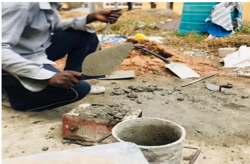
Figure 3: Casting of the concrete cubes
