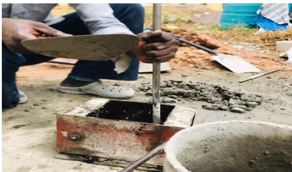
Figure 4: Compaction of fresh concrete with tapping rod
