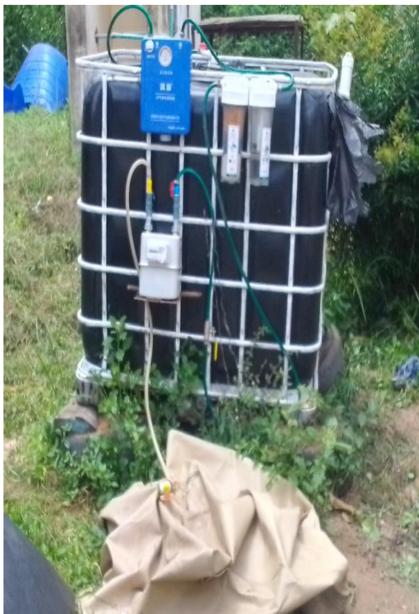
Plate.1: Assembled biogas plant
