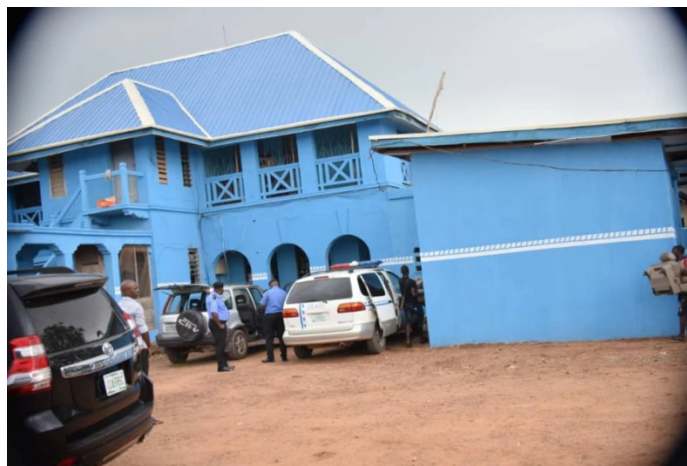
Plate 8: Front View of the FRSC Headquarters, Abeokuta
