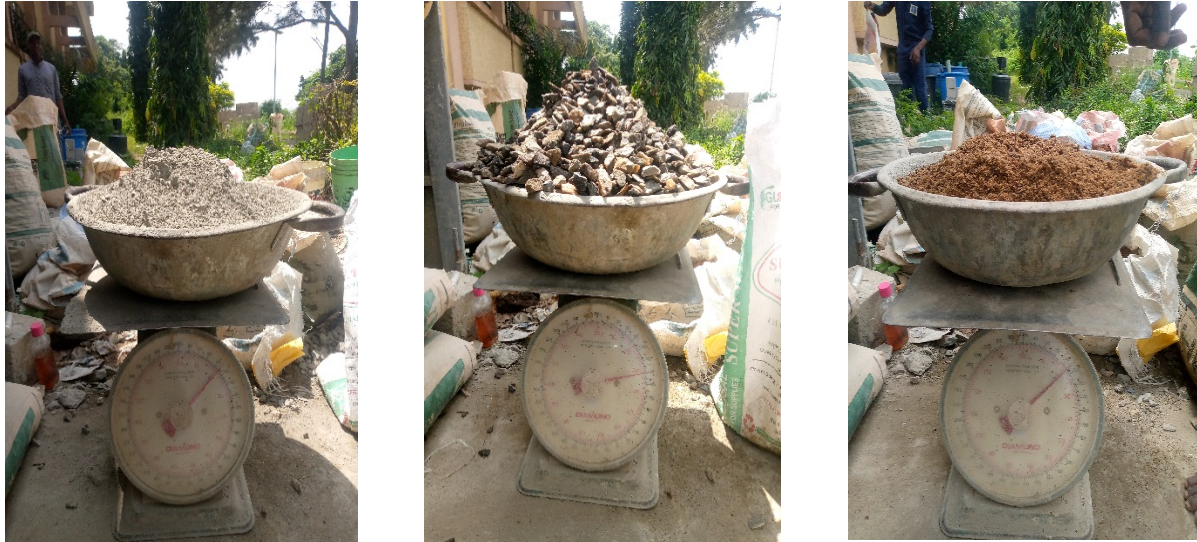
Plate 2: Concrete Constituent Batching by Weight
